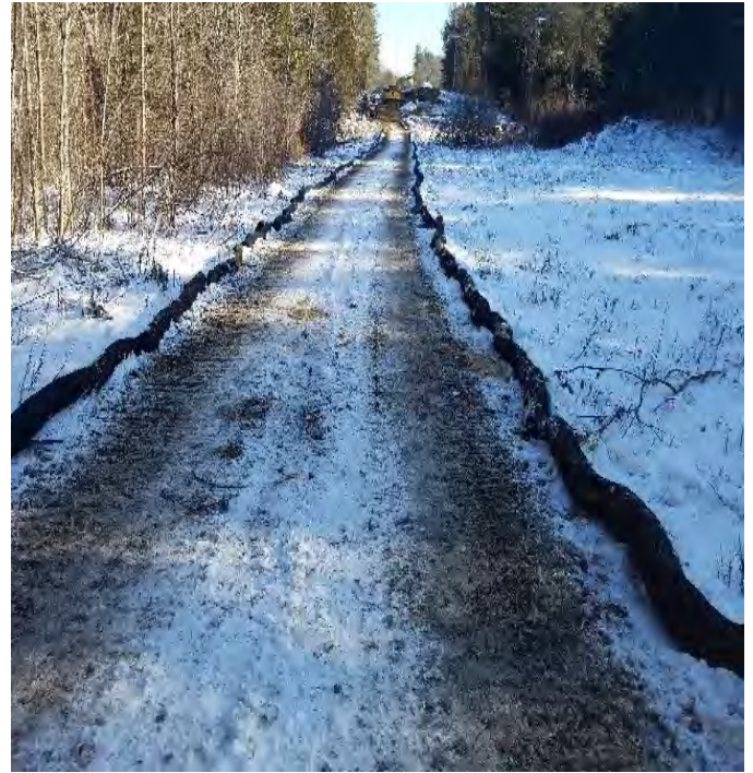
Fig 6: Access road through wetland DW33, heading to Str. 55. Viewing east. (12-19-19).
