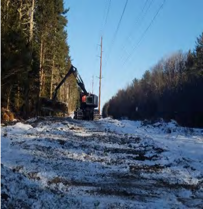
Fig 1: Removing timber mats on access road between Strs. 16-22. Viewing north. (12-19-19).
